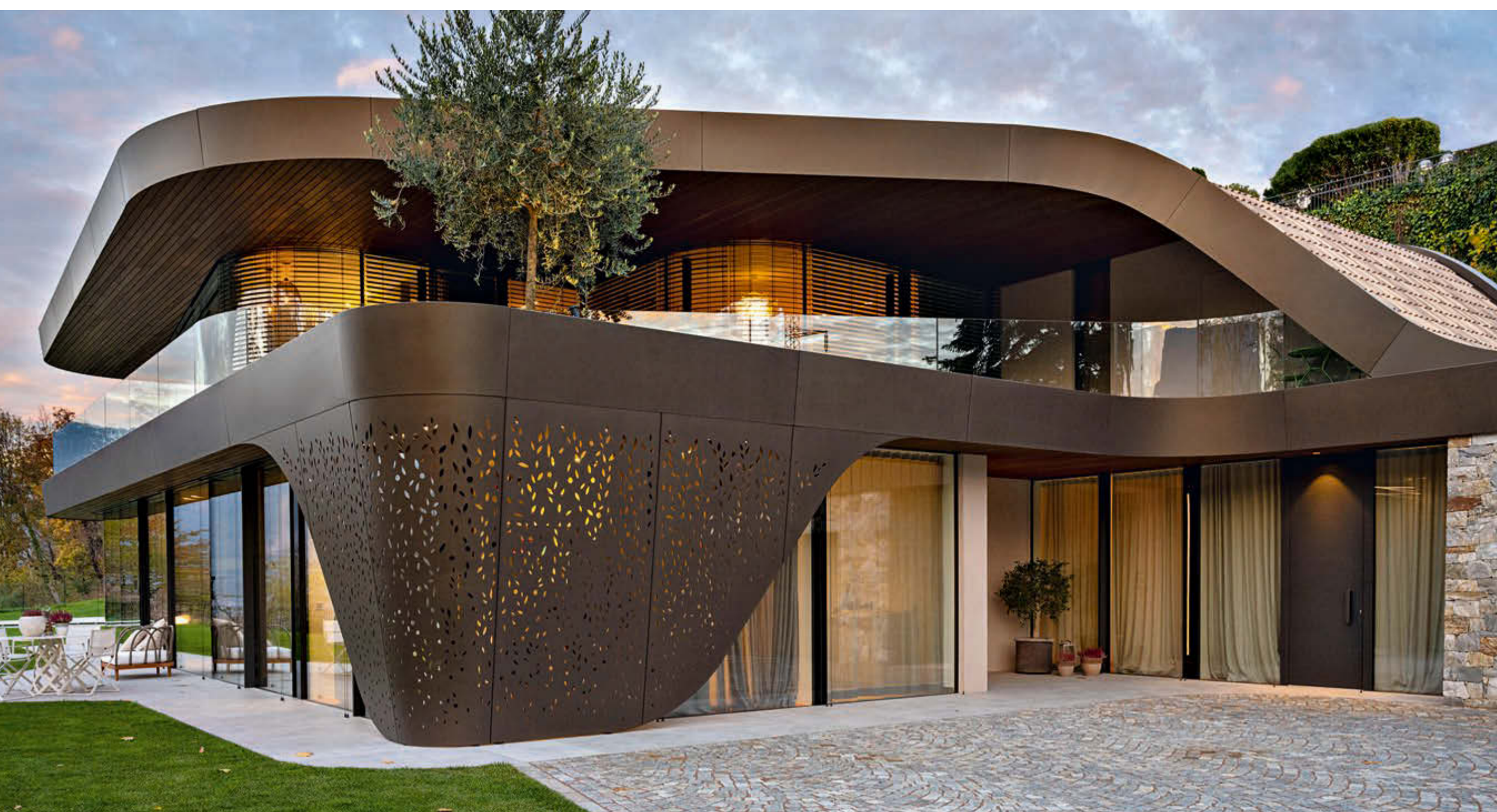
With its large glass areas and protective sheet metal elements, the building envelope offers transparency and privacy alike.
