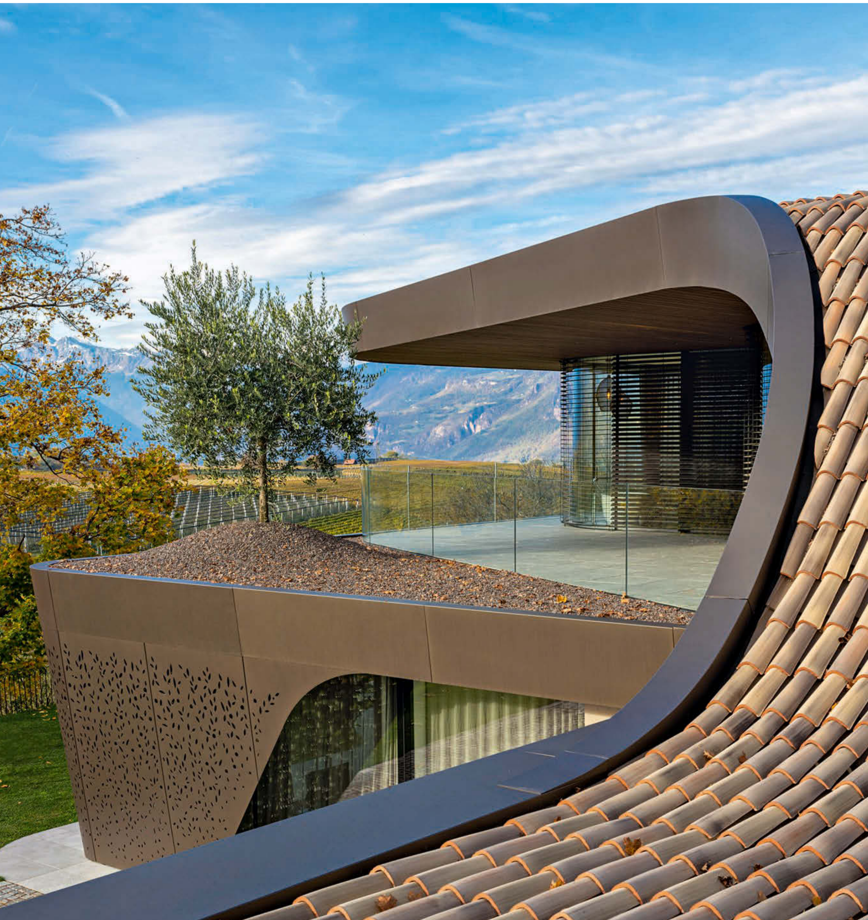
Following the extensive renovation, the curved roof, large windows and carefully selected material characterise the Villa EB.
