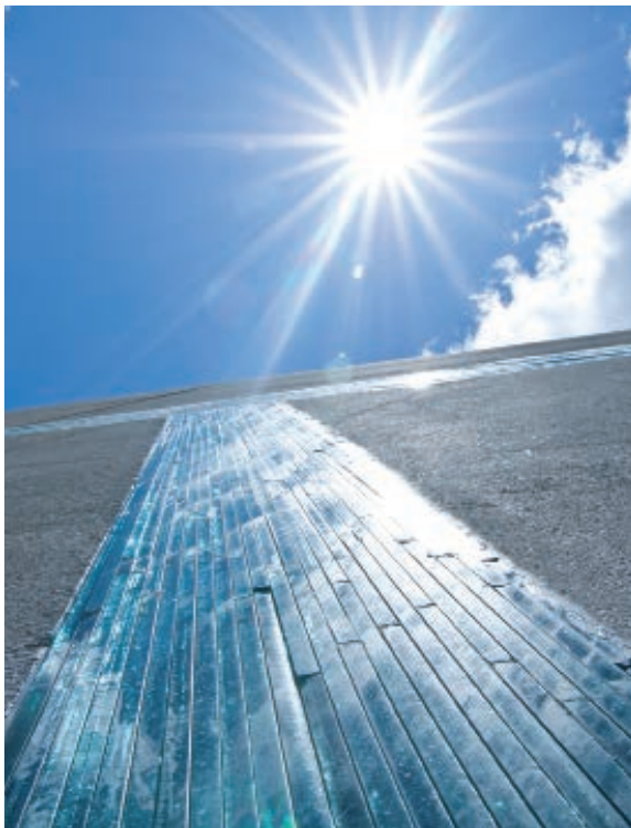
Glass bands embedded in wall
