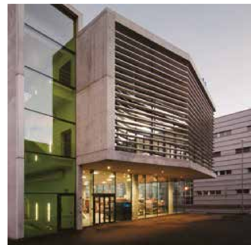
从外面即可看出内部清晰的区域划分 Clear and formal internal division be perceived already from the outside
